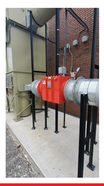
The VigiFLAP is similar to a No Return Valve, but is much more flexible in its application as it can be installed in either a horizontal or vertical position. Available in diameters from 6" up to 52". Both devices come with a micro-switch for system shutdown, a dust level sensor, and a separate control panel. Both these products are essential to an NFPA compliant dust collection system, and can be paired with other ATEX certified devices and accessories.
