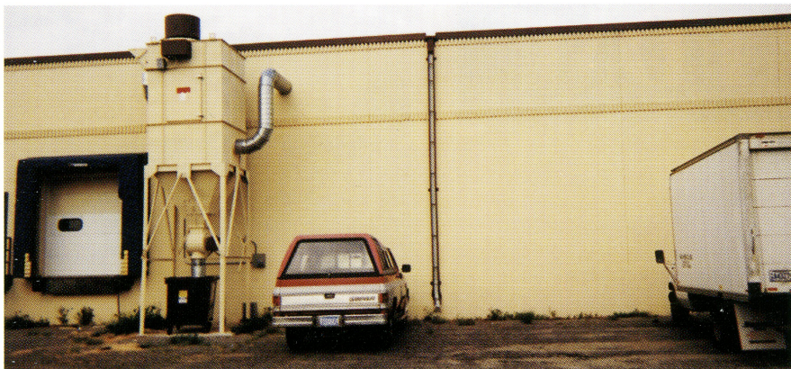
The Mal-O-Sen facility has been rebuilt, and the same dust collector stands outside the new building.
